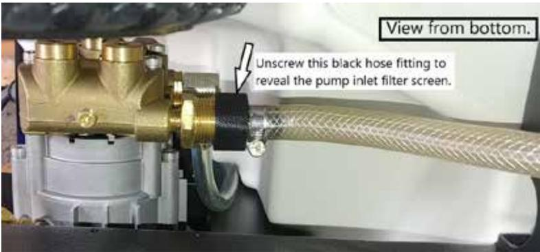
Figure 10 – Location of pump filter screen.
