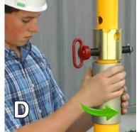
Rotate the Threaded Locking Collar to snug the Load Plate of the Jacking/Shoring Post up against the Load [see green arrow].
