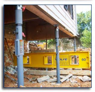
Left, Jacking/ Shoring Posts provide temporary overhang support.
