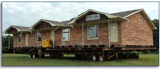
Above, and Below Left, Jacking/Shoring Posts provide safe temporary support for the porches and overhangs during subsequent Lifting and Transport operations.
