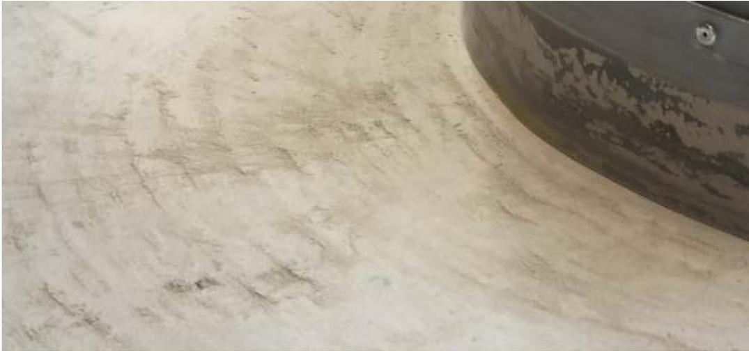
On 25” Grinder, make sure the planetary is spinning, especially throughout the heavier grits. Hitting things or grinding excessive transitions can cause the planetary belt to tear. Extra belts are included and easily replaced by removing cover on bottom side of grinder between the 3 heads.
