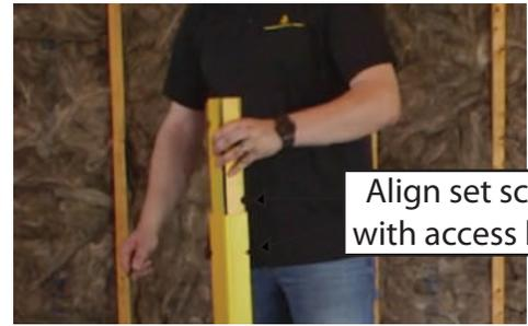
Align set screws with access holes.
