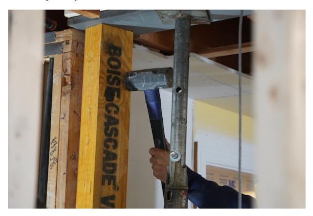
**Tip:** Cut the posts 1/8" long and then gently driven into place by tipping the bottom of the stud in place and then drive the top along the beam surface. It should not take a lot of force to drive them in place, if it does remeasure and recut.
