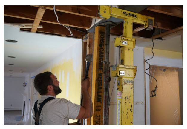
The Sumner Roust-A-Bout lifts enables one man to lift and place loads in tight locations that would be impossible with other lifts. One lift can raise a 1,500 lb. load to heights up to 25-feet in minutes.
