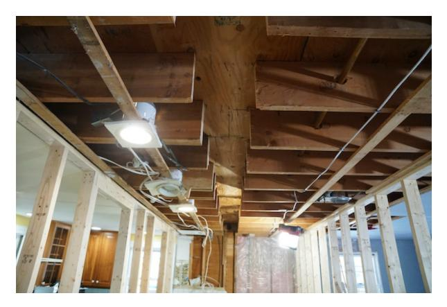
We used a Bosch Green line laser to connect both beam pocket locations and then used a speed square to mark cut lines directly on the joists. To start each cut, a circular saw was used and finished up with a reciprocating saw.
