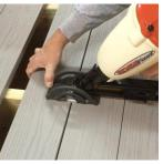
Place the tool gap spacer against the loose edge of the decking that is your starting board. Slide the next board up to the other side of the gap spacer. Now the spacer should be between the two boards. Pivot the tool down so that the magazine is parallel over your starting board. While pulling the loose board tight to the spacer, push the tool down towards the base and oncoming board. The
